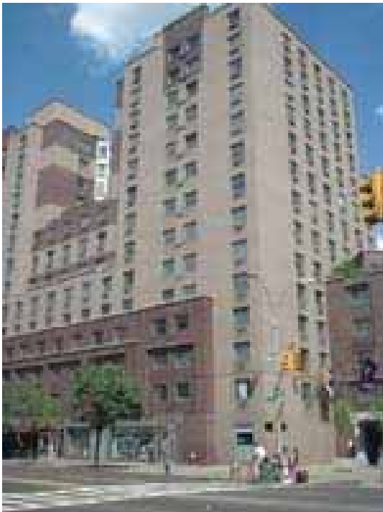
Third Avenue North Dormitory (1986) 75 Third Ave 337,600 sq. ft.
